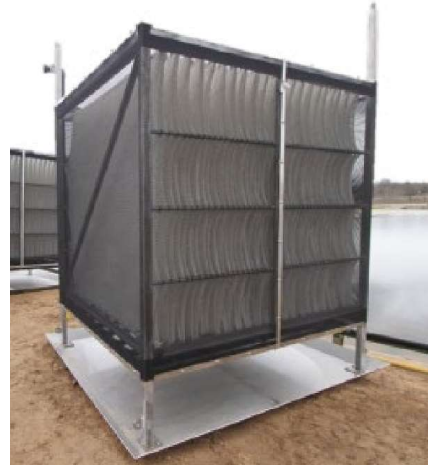
Photo 1: Lagoon Intensification Fixed Film Media
