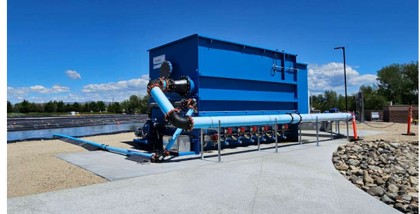
Figure 1: Cloth Disc Filter Tanks
