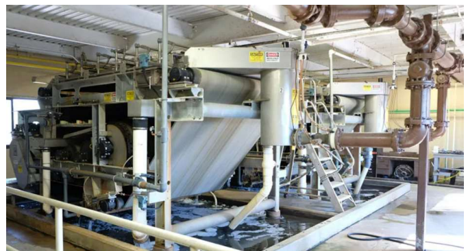
Photo 2: Example Belt Filter Press for Solids Dewatering
