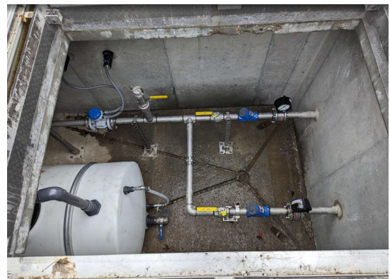
Figure 2: Typical lift station valve vault
