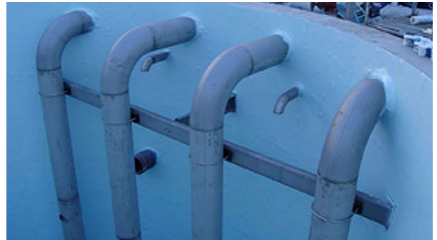
Figure 1: Lining systems on concrete structure
