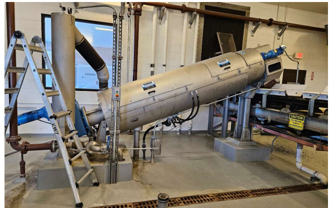
Photo 1: Example Screw Press for Solids Dewatering
