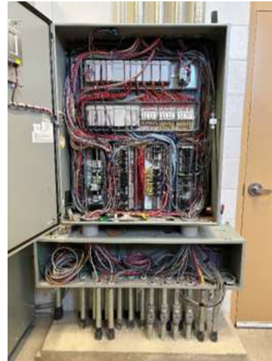
Photo 1: Headworks PLC Cabinet
