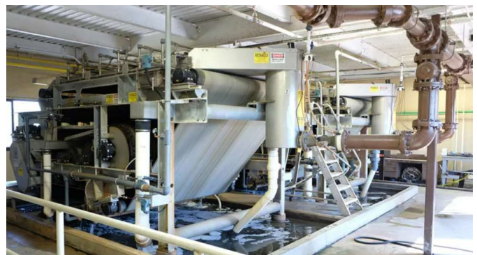
Photo 2: Example Belt Filter Press for Solids Dewatering
