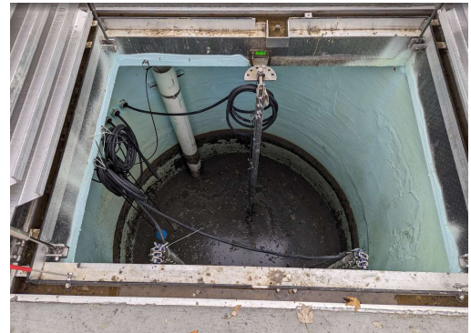
Figure 1: Lining systems on concrete lift station
