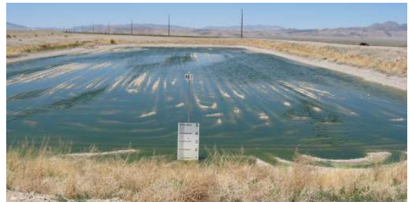
Photo 2: Example of a flooded Infiltration Basin
