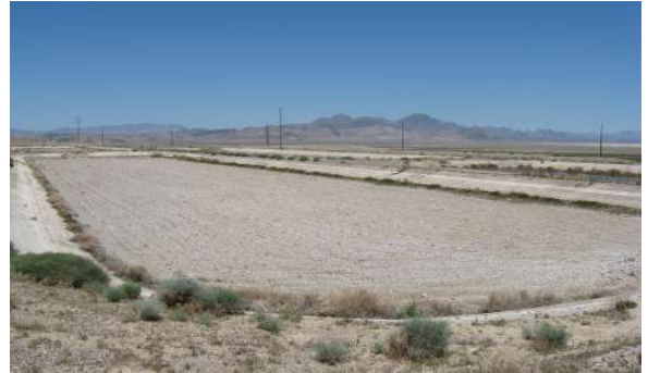
Photo 1: Example of a Dry Infiltration Basin
