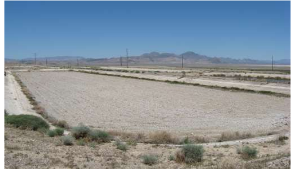
Photo 1: Example of a Dry Infiltration Basin
