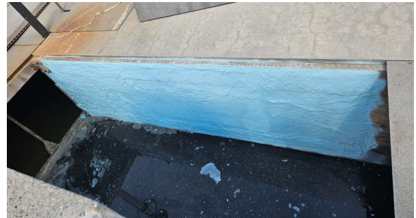
Figure 2: Concrete Channel Coating Example
