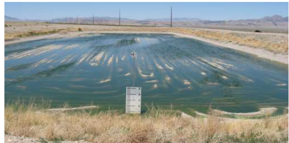
Photo 2: Example of a flooded Infiltration Basin
